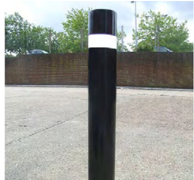
Bollard with retroreflective tape
