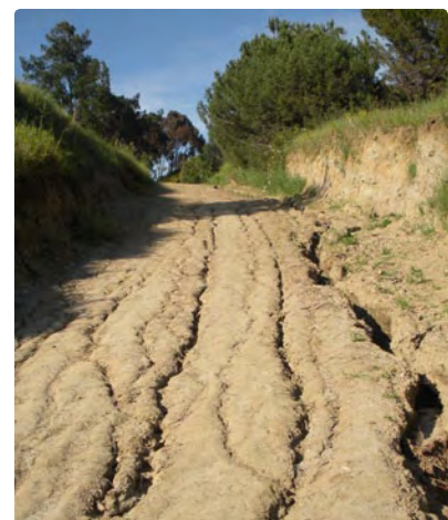
Fall Line trail in Kenneth Hahn State Recreation Area has resulted in a significant amount of trail erosion.
